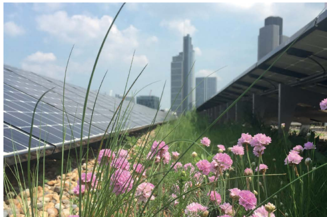
Source: Dusty Gedge: Solar Green Roof, Standard Chartered, London
